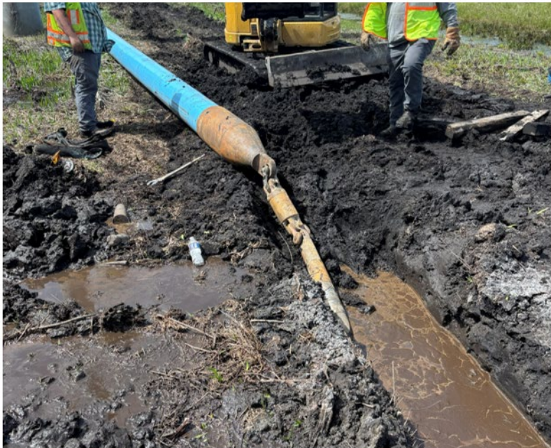
Photo-2: Sandy's-Hauling-connecting-pipe-to-drill-rod-at-STA-52+56.03.
